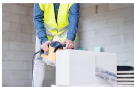
SAFETY BLOC<sup>®</sup> PRIPREMA ELEMENATA NA MJERU
